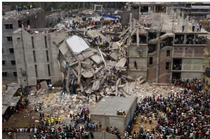
Fig. 16. Savar Rana Plaza building collapse (New Age Online, 2013).
